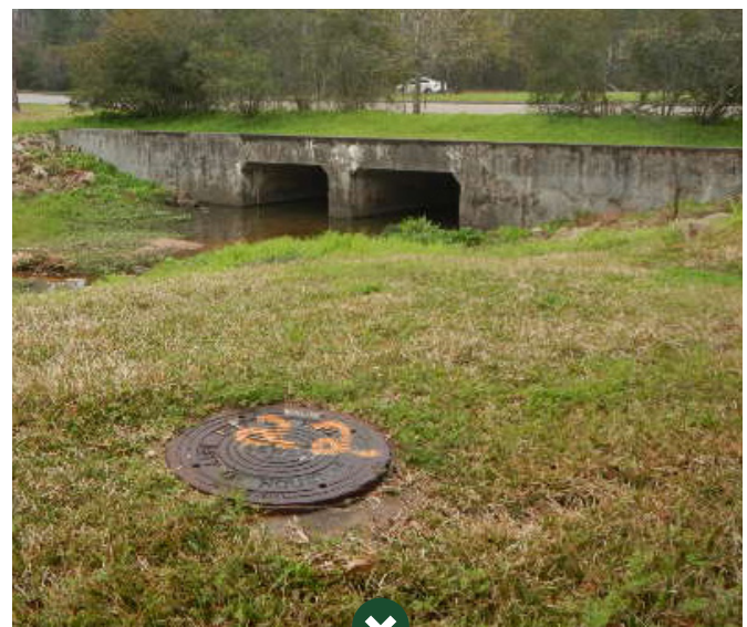
Completed installation from outside of manhole.
