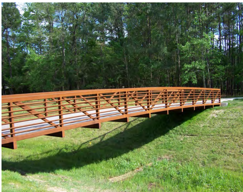
Figure 7.1 Existing Pathway Bridge
